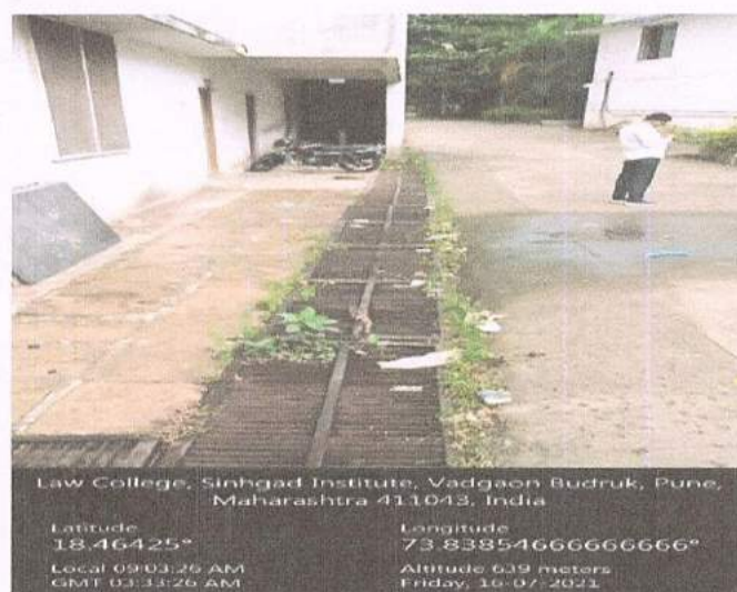
Photograph of Rain Water Harvesting Channel:
