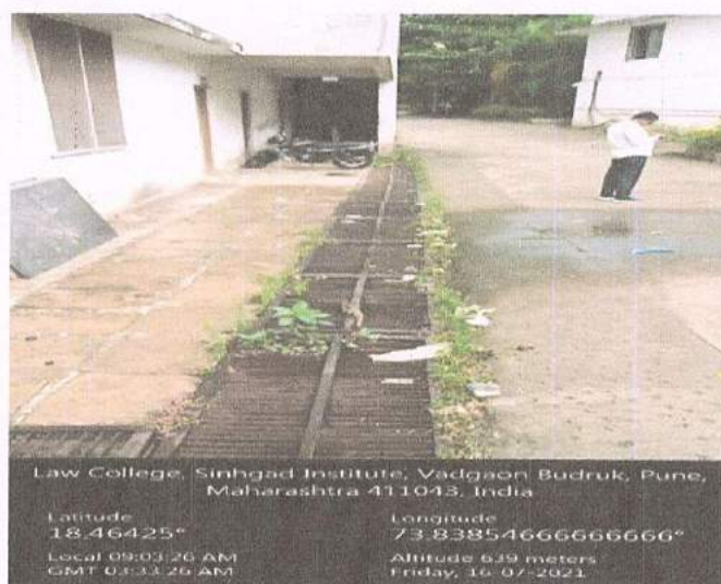
Photograph of Rain Water Harvesting Channel:
